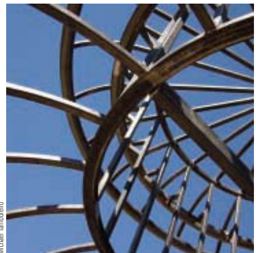
Below: A tangle of precisely curved steel tubes, pipe and bar stock comprise the cap structure.
